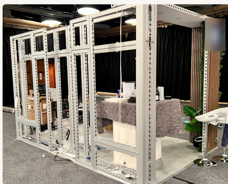
Bare frame: 62mm-grid profile at build-up
