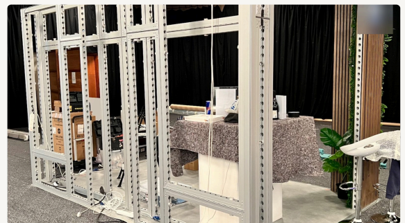
Bare frame at build-up, showing the 62mm-grid profile, split-height walls and the beam-support post.
